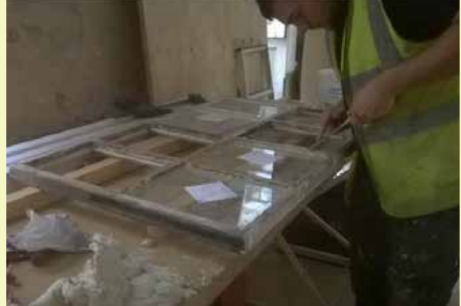
Window repairs underway at Croome Court © NT Croome
