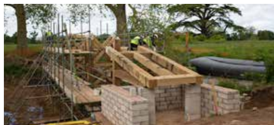
Chinese Bridge under construction © James Dobson
